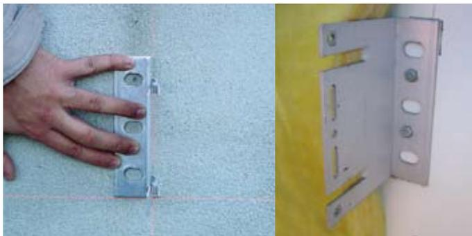
Trace the axis for positioning the vertical profiles, separated by distances depending on the size of the terracotta products and on the width of the vertical joint. Fix the brackets with anchors on both sides of the future position of the profile. Fix the insulation around those brackets.
