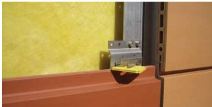
Insert the clips on the profiles. Install each product, one above the previous one, on 2 clips below. Screw the 2 clips above, positioning them by respecting a distance above the previous clips or by using spacers above the terracotta.
